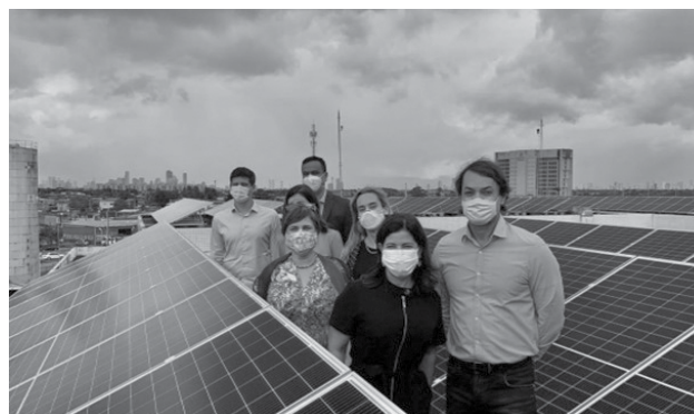
Figura 11. Leta Vieira (ICLEI) and the Recife City Hall team in through the installed photovoltaic system. Photo: Recife City Hall
